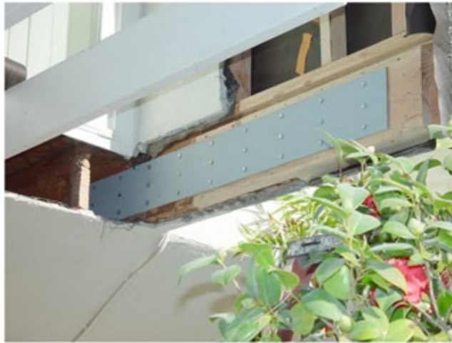
Photos above to left and right show 2nd layer of steel reinforcing brackets on double rafter. The 2nd bracket was five ft. in length. All steel and wood was primed on all six sides PRIOR to install, except for wood encased within the stucco structure, which is protected by moisture barrier paper.
