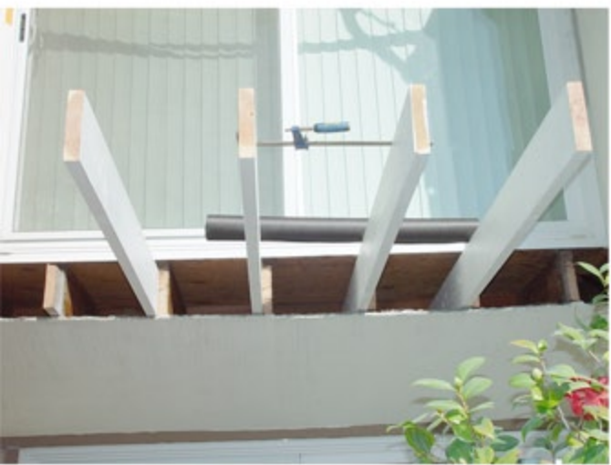
Photo above left shows most but not all new rafters installed, and before fire blocking was installed between, followed by moisture paper, metal lath, and three separate coats of stucco.
