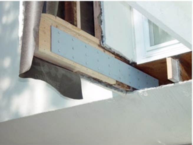
Photos above to left and right show 2nd layer of steel reinforcing brackets on double rafter. The 2nd bracket was five ft. in length. All steel and wood was primed on all six sides PRIOR to install, except for wood encased within the stucco structure, which is protected by moisture barrier paper.
