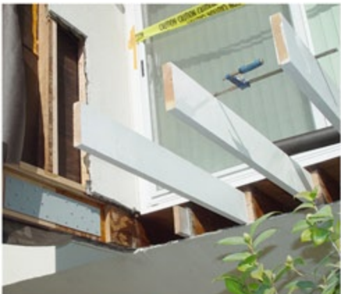
Balcony Reconstruction Project. Photos to left and right show partial new rafter installs, first layer of steel reinforcing brackets, and replacement of vertical wall studs both sides.
