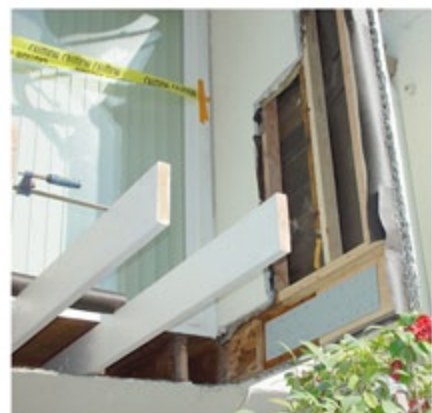
Balcony Reconstruction Project. Photos to left and right show partial new rafter installs, first layer of steel reinforcing brackets, and replacement of vertical wall studs both sides.
